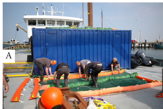
Figure 30. Preparation of the artificial seagrass on the ship. Photo RCE Maritime Programme (A). The artificial seagrass is deployed on the wreck. Photo RCE Maritime Programme/ Paul Voorthuis (B).
