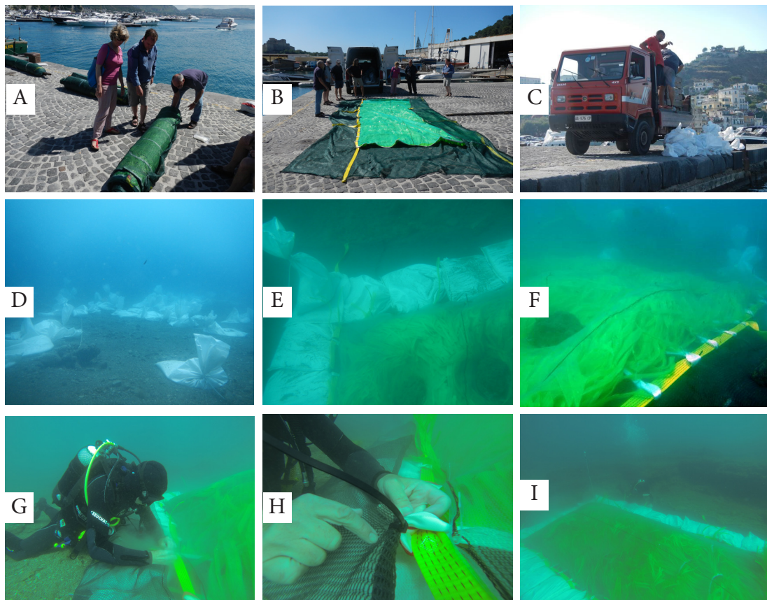
Figure 39. Arrival of the mats (A,B). Placing of the sandbags (C,D,E) Installation of the mats (F,G,H,I). Photos ISCR and The National Museum of Denmark.
