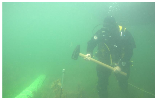
Figure 33. Diver hammering a seagrass anchor into the seabed. Photo Viking Ship Museum.
